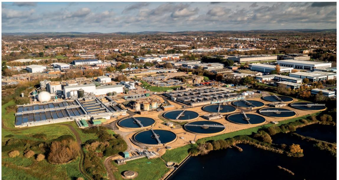
Budds Farm Wastewater Treatment Works.
