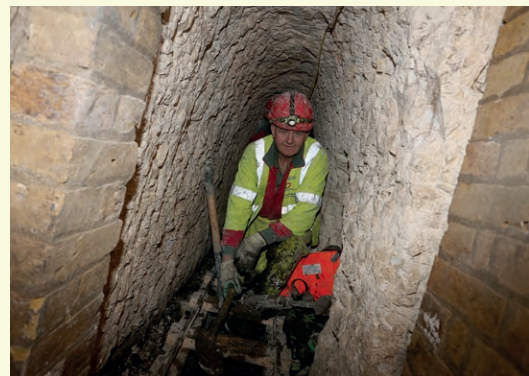
Upgrading the sewer adits at Thanet.
