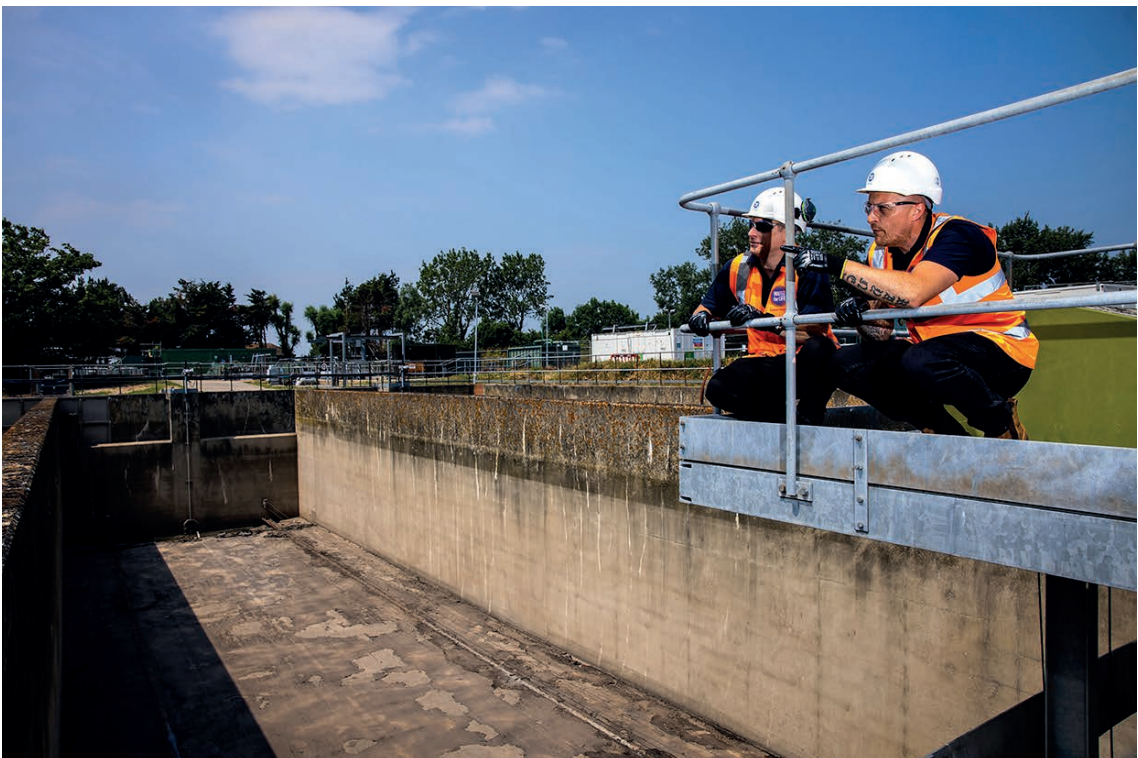
Inspecting the Swalecliffe system
