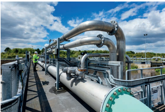
Peel Common Wastewater Treatment Works
