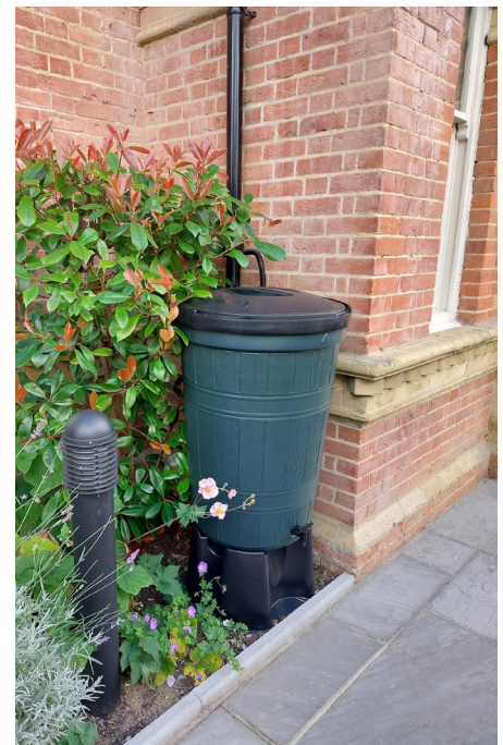
Installed slow-drain water butt in Havenstreet
